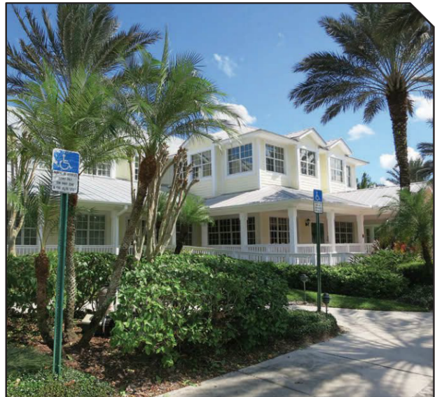
Beyond cutting down on maintenance costs, Treasure Coast Hospice more importantly was able to reduce the risk of hospital acquired infections by installing UVGI systems on its AC and PTAC units.
